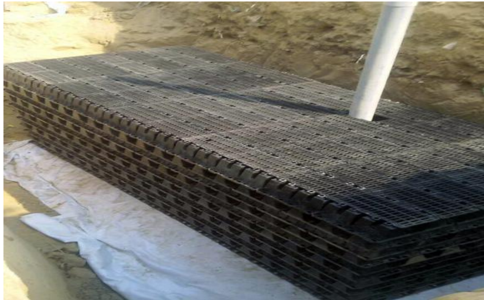
TYPICAL SECTION OF CROSS WAVE POLYMERS
