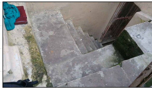
MICROBIOLOGICAL GROWTH AND DAMAGED FLOOR
