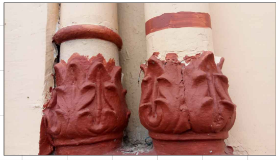
DAMAGED ELEMENTS, CRACKS ON THE ELEMENTS, MISSING ELEMENTS
