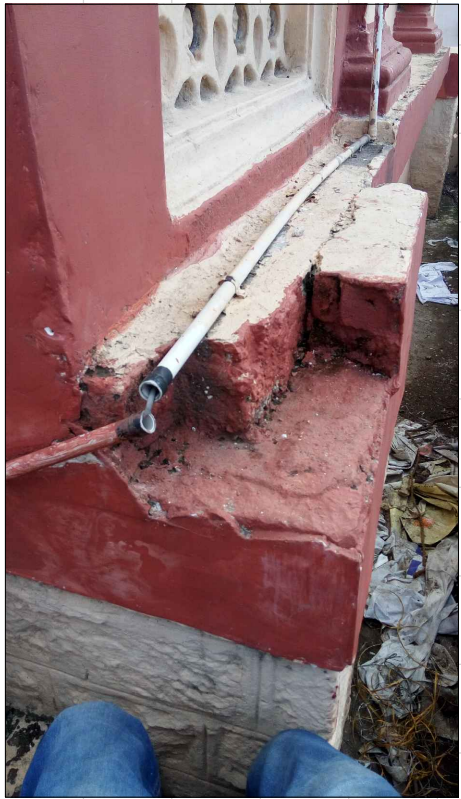
DAMAGED ELEMENTS ON PARAPET, CRACKS SEEN
