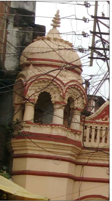
MISSING ELEMENTS ON THE ARCH i.e. THE FLOWER MOTIFS AND SOME ELEMENTS ARE DAMAGED TOO
